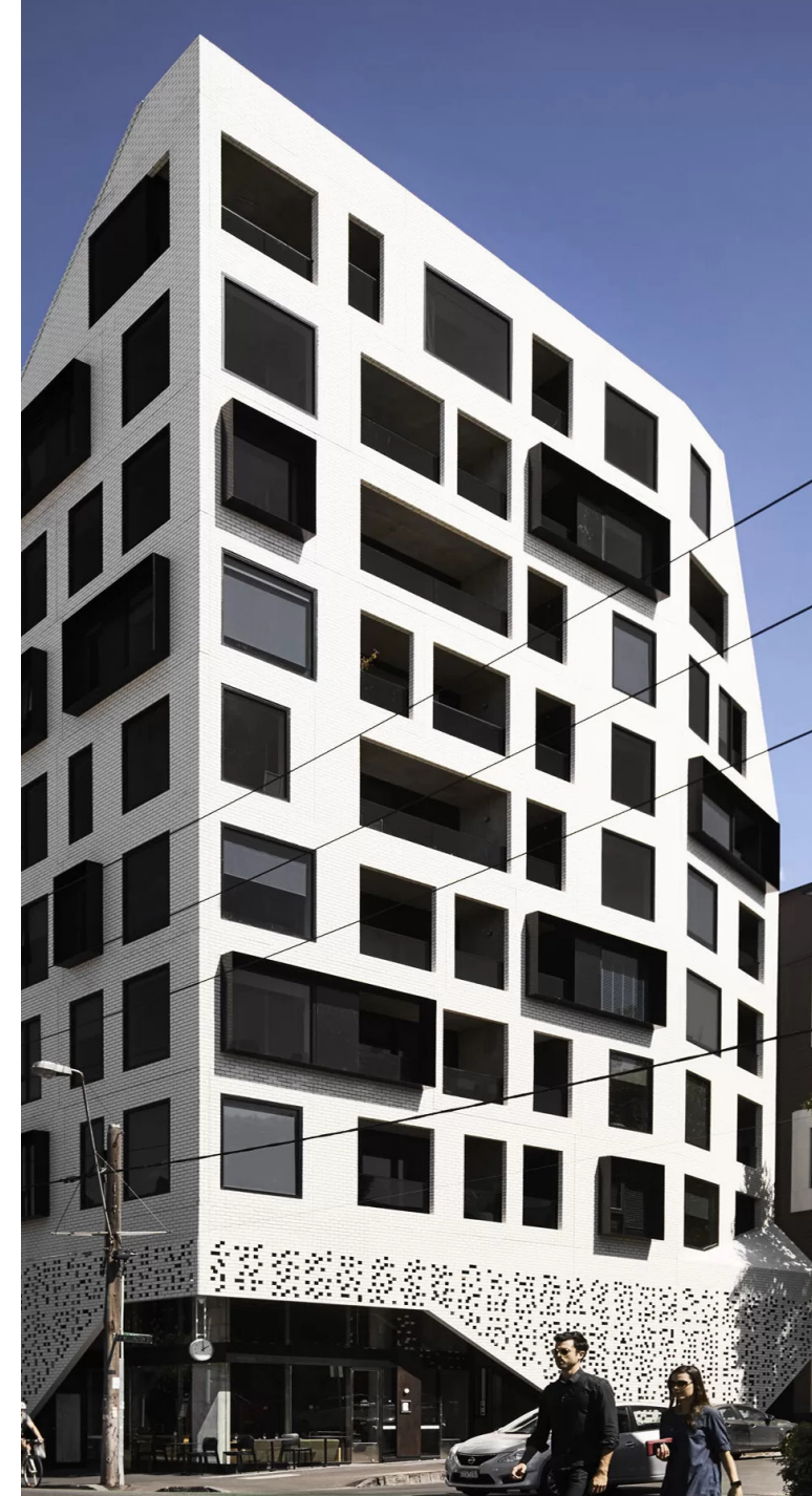
Figure 25. Peel Street, Melbourne, DKO Architects (Source: DKO Architect)
